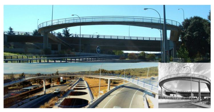
The Zarzuela Junction is located on the M-40 belt motorway, over the El Pardo motorway and the River Manzanares, connecting the M-40 and M-30 belt motorways with the El Pardo motorway. Concentrated in a very small area, there are 2,247,20 metres of viaducts and bridges and 32,760 m2 of structures.
